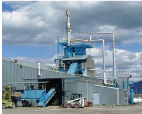
EPI Pilot Plant
