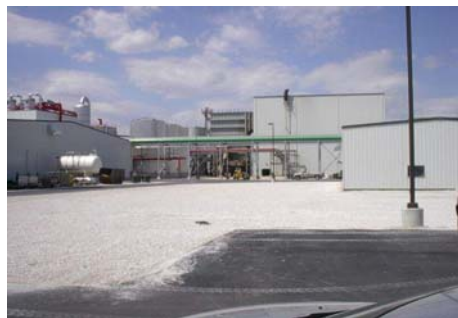
Lincolnway Energy - Nevada, IA 220MMBtu/hr - PRB Coal - 2006
